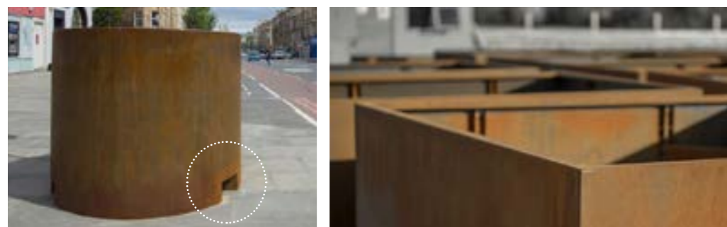
Forklift slots fabricated for mobile planters/additional flexibility
