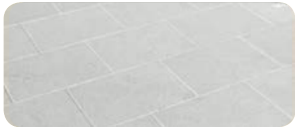
Concrete Flag paving
